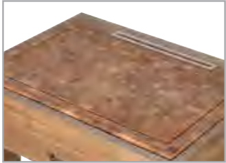
The above photo shows NVW041 block top.
